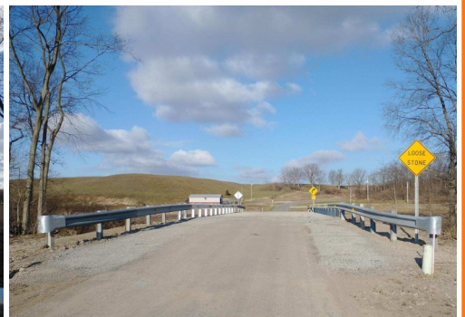
Completed new bridge
