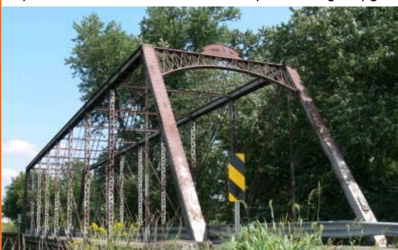
Historic bridge BR 21-1.01B
