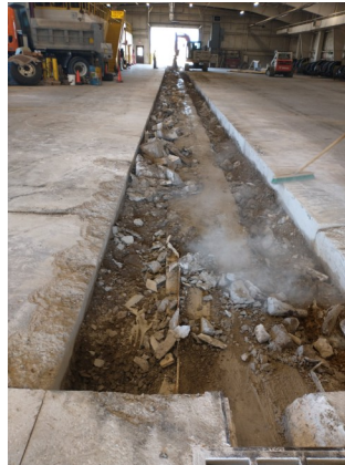
Old trench drain cut out
