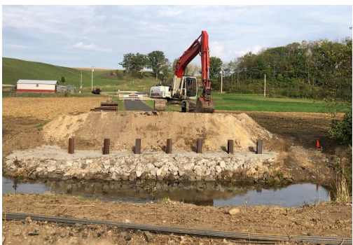
Piling set; ready to form abutments
